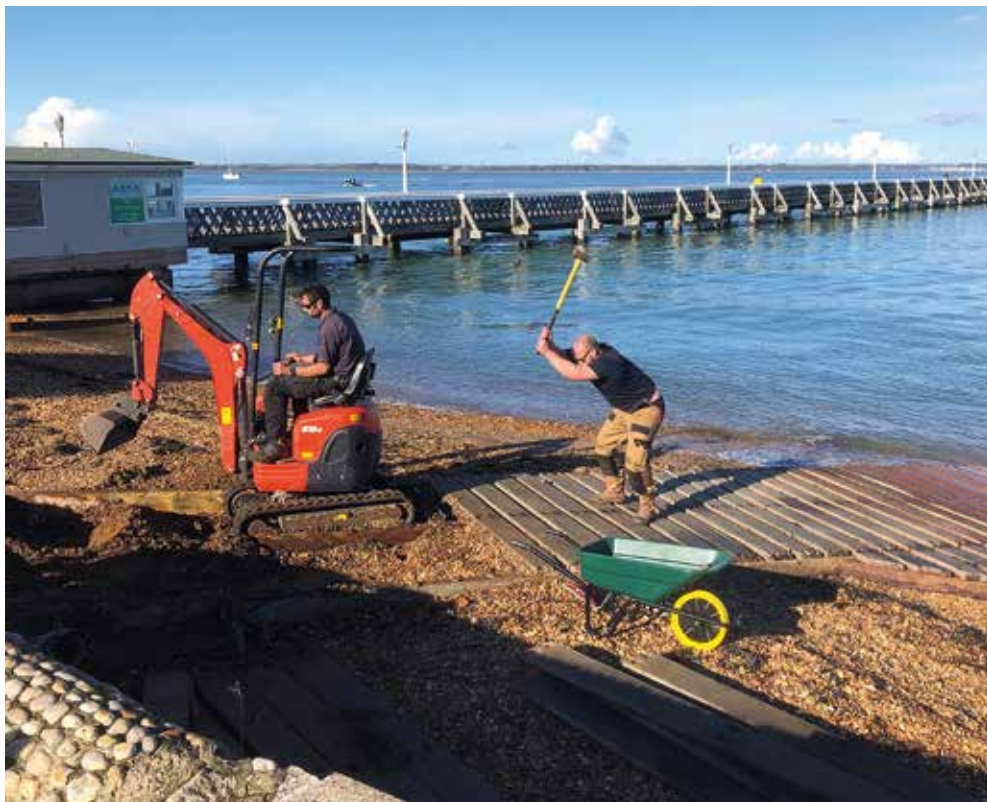
The slipway being cleared for refurbishment
